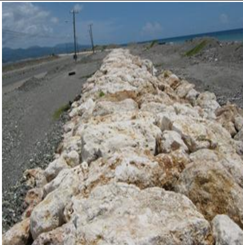
Revetment on the side to the Caribbean Sea, due East
