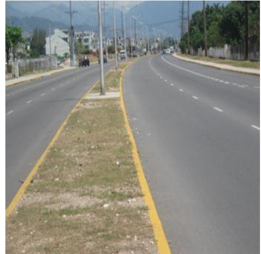
A section of the newly constructed Washington Boulevard
