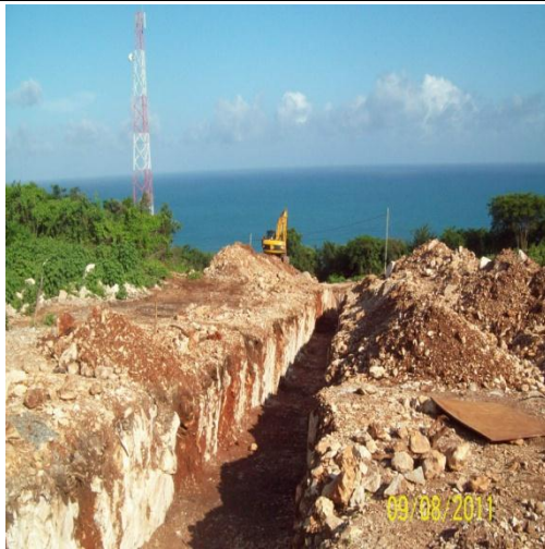
Excavation Activities on Creighton Hall Infrastructure Development
