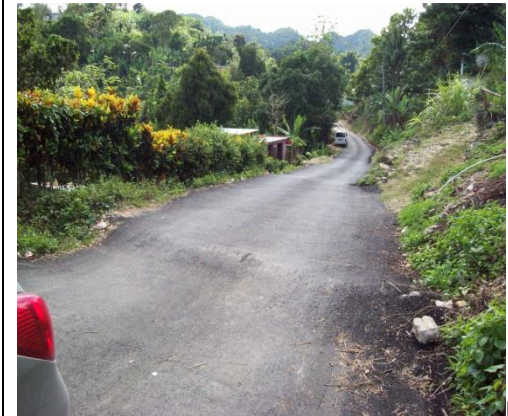
Road with asphalt overlay and cross-drain
