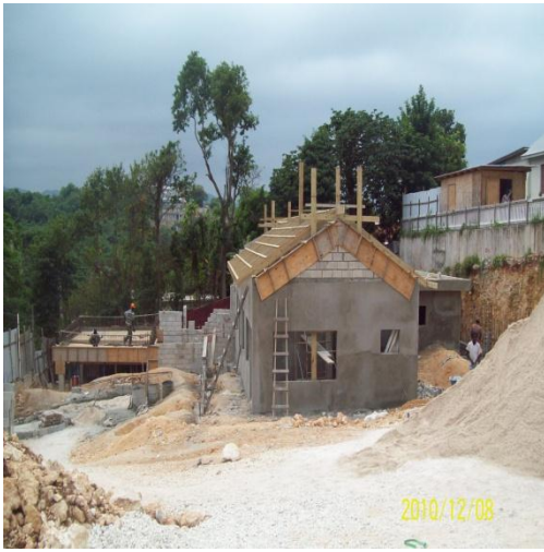
Project During Construction
