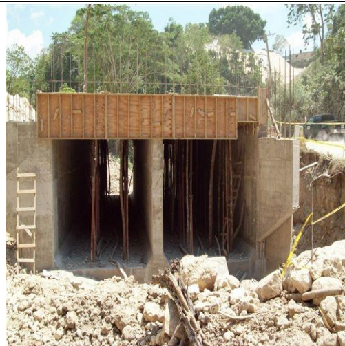
Reinforced Box Culvert under construction
