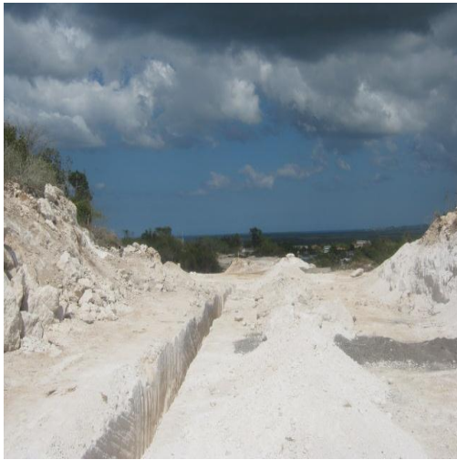
Excavation for Lateral Sewer Pipes - Sector A
