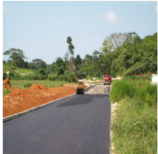
Paving Operation within the Infrastructure Works
