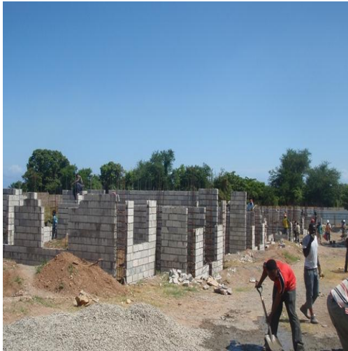
Initial stages of Construction
