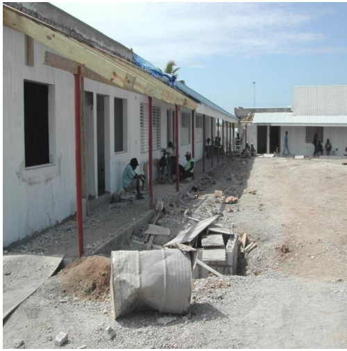
View of Site on April 12, 2011
