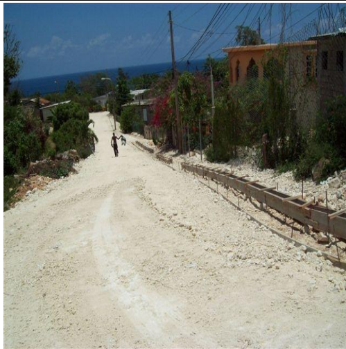
Initial stages of road works
