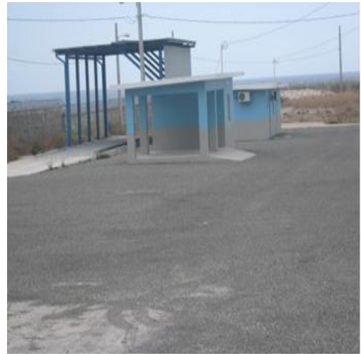
Completed Truck Scale Facility
