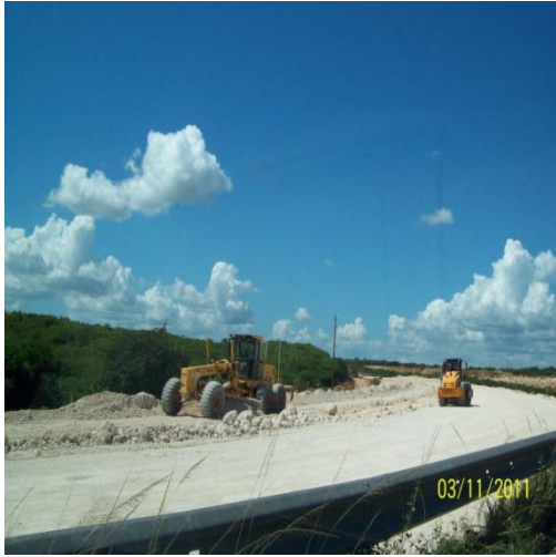
Road Construction Activities at Sandy Bay, Clarendon
