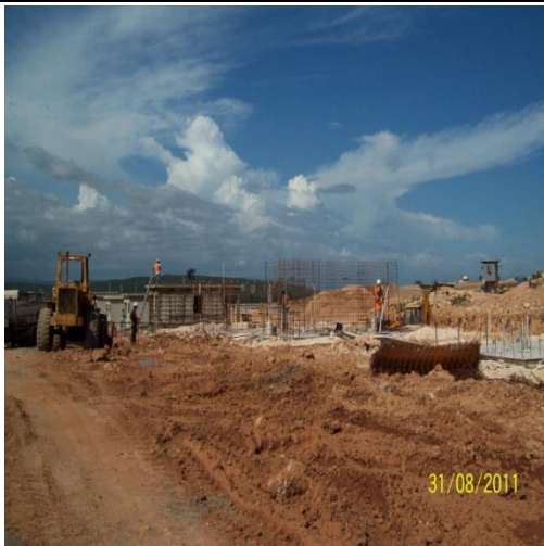
Construction of Housing Units
