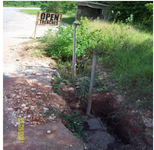
Testing of Pipe Lines
