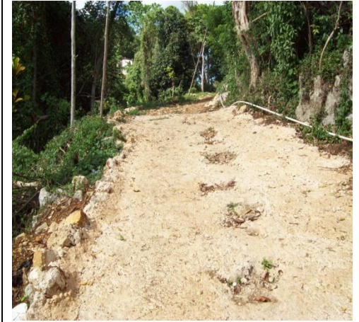
Concrete overlay on lane
