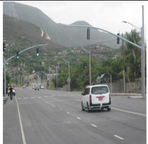
Section of the Dry River Bridge and Rehabilitated Roadway
