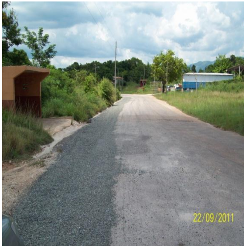
Permanent Reinstatement of Excavated Pipe Lines
