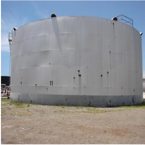
View of Existing Tank No. 11 as at December 2011
