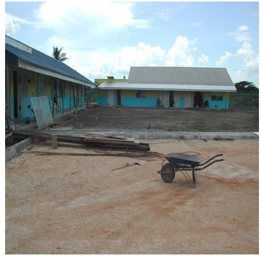
View of Site on October 6, 2011
