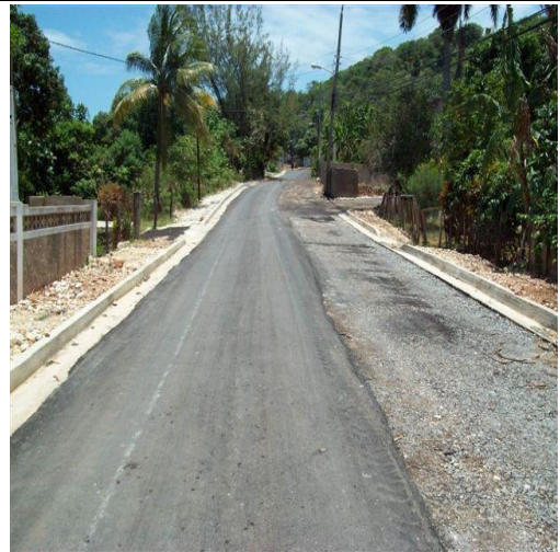
Road partially paved
