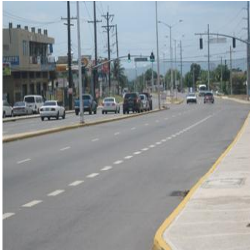
One of the intersections along the newly constructed Washington Boulevard
