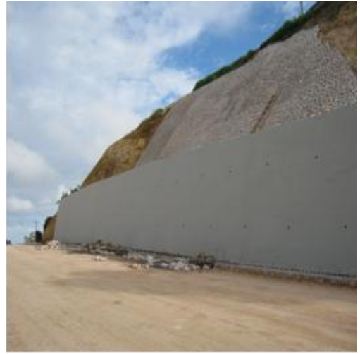
One of the Retaining Walls
