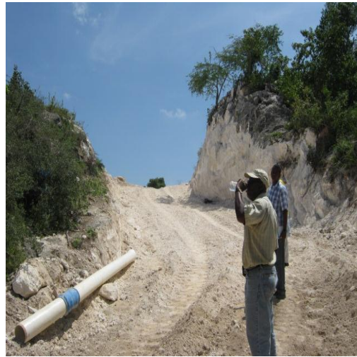
Road Cut - Sector A
