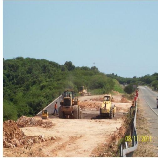
Bridge Construction Activities at Sandy Bay, Clarendon
