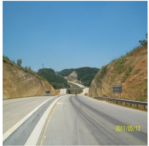
Completed Section of the Toll Road
