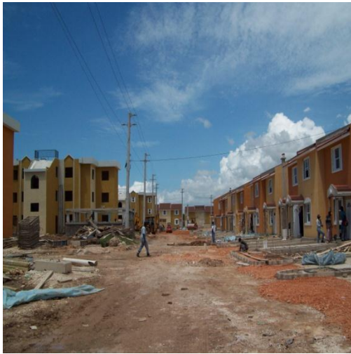
Construction Activities being undertaken
