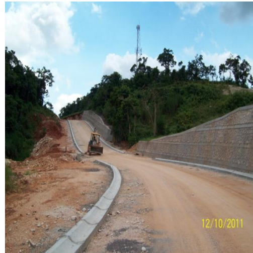
Completed Retaining Wall and Kerb Walls
