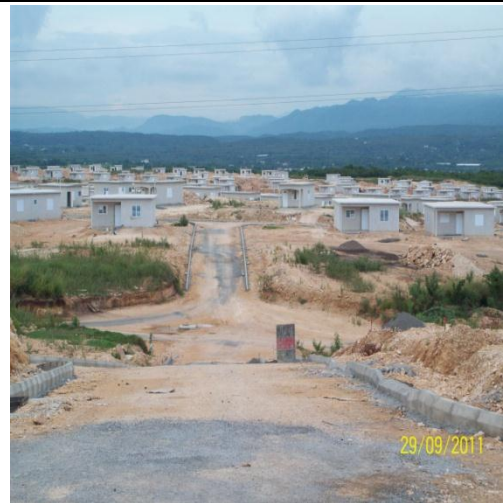
Completed Housing Units
