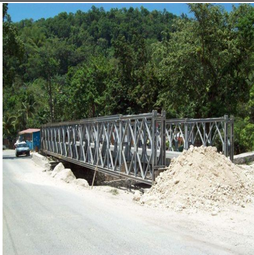
Bailey Bridge at John's Hall
