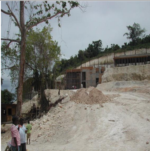
Progress of works as at September 2009
