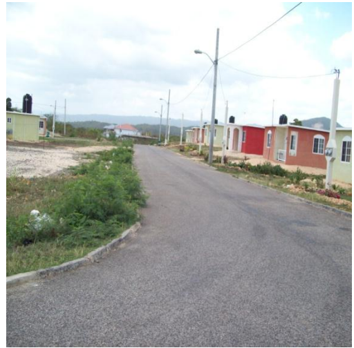
Completed Housing and Infrastructure Works
