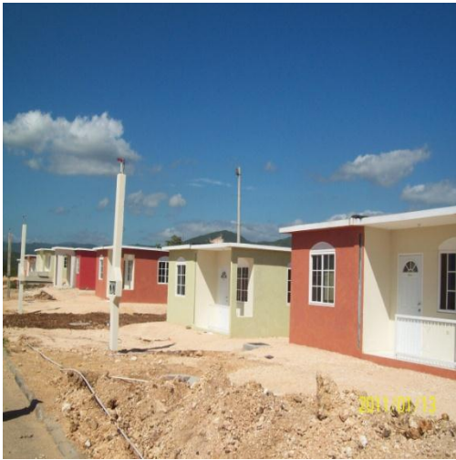
Completed Housing Units
